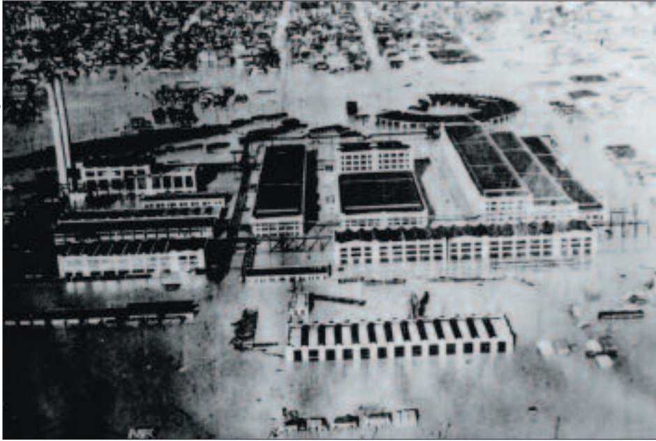
This aerial shot of the Illinois Central Railroad's huge Paducah shops shows the extent of the devastation.
