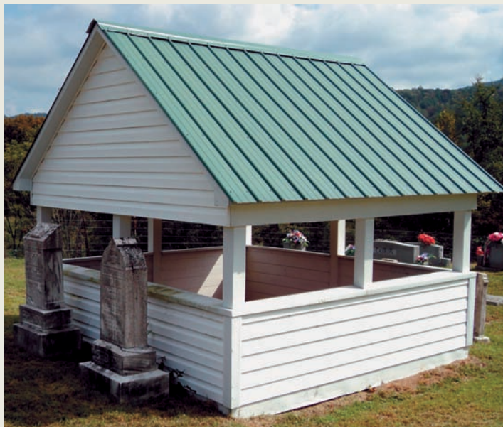
The grave house for William (1845-1922) and Mary J. Brown (1848-1930) is one of two examples found in the Pleasant Hill Baptist Church in Sunnybrook, Wayne County. Both grave houses have recently been reroofed and covered with aluminum siding.
