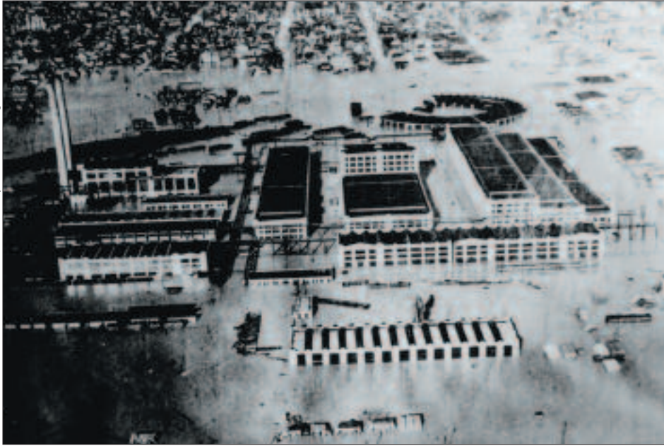
This aerial shot of the Illinois Central Railroad's huge Paducah shops shows the extent of the devastation.
