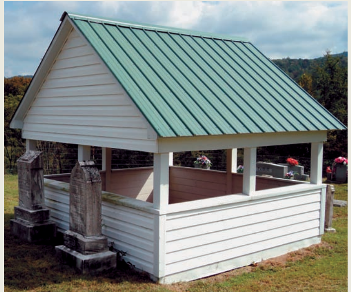
The grave house for William (1845-1922) and Mary J. Brown (1848-1930) is one of two examples found in the Pleasant Hill Baptist Church in Sunnybrook, Wayne County. Both grave houses have recently been reroofed and covered with aluminum siding.
