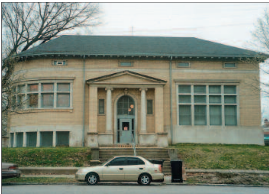
The Portland Branch of the Louisville Free Public Library is distinguished by its curved corner.
