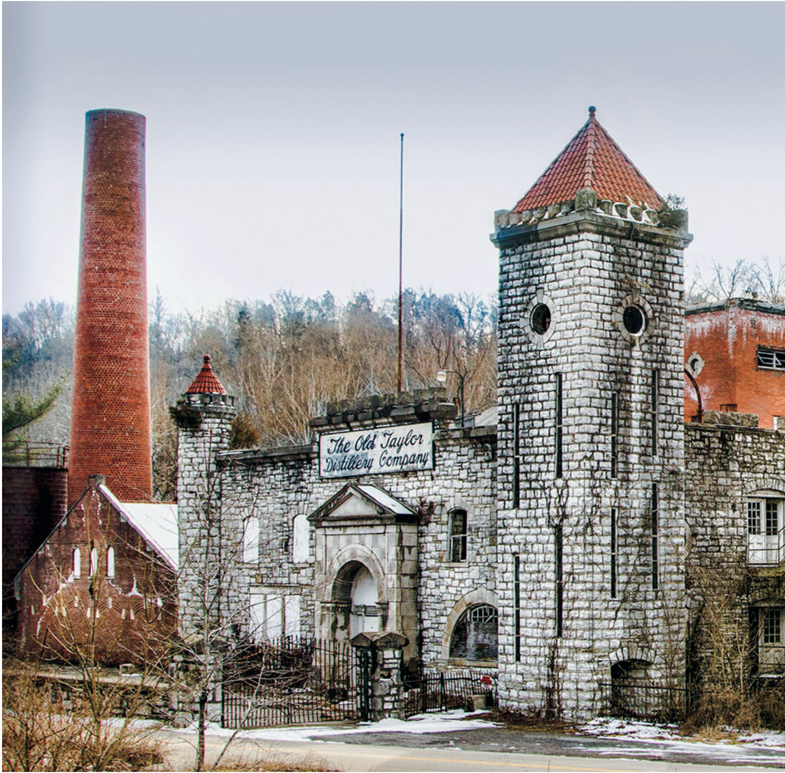
Old Taylor Distillery, Woodford County. A full view of the distillery shows the lengths that Taylor went to to create his distillery castle. The main attraction is of limestone block; the oven house to the left and offices to the right are of brick. A grain house is in the far right corner, and the water tower, with its crenellation, is in the middle background.
